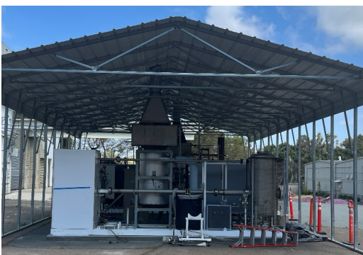
Figure 4. Picture showing the General Atomics iSCWO system on-site.
